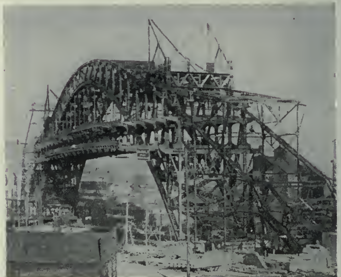
Fig. 4—Archclosed and double-deck floor steel placed by returning Travellers.
